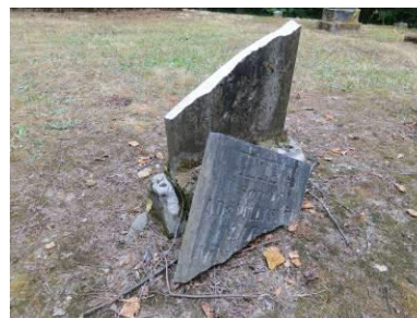
Marker 04.16 had a very fresh break which is an ideal time to repair as it has not yet had time to weather. In this state, the repair can be made practically invisible.
