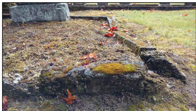
Example curbing deterioration in the cemetery.
