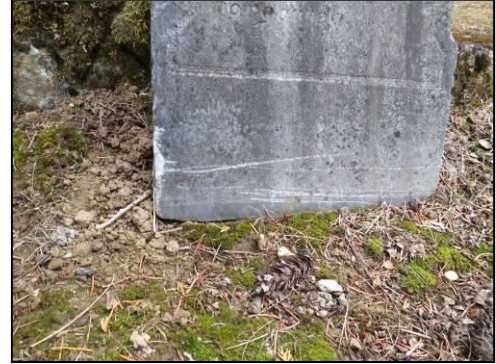
The George L. Alderman headstone is off its base and has subsequently been struck repeatedly by string trimmers (#05.11).
