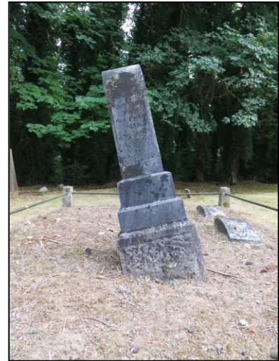
Marker 09.23 was leaning at 12 degrees. It was releveled as part of this project in September 2017.
