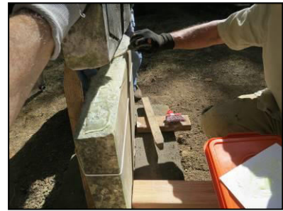
Carefully applying epoxy, keeping it well back from the edges and only where the two stones will touch.
