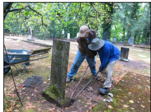
Often leveling takes no more than a stout pry bar and some gravel. Other times the weight is too great and a tripod is needed. Stone is heavy – figure 200 pounds per cubic foot to be on the safe side.
